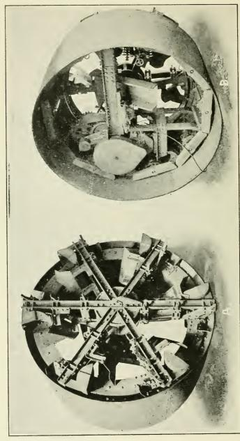
(A) Front view. (B) Rear view. (From Fig. 78.—The John Price rotary cutter in a small shield to work in London clay. Trans. Am. Soc. C. E., vol. 54, Part F.)
