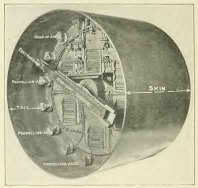
Fig 83.—The parts of a shield. Rear perspective.
