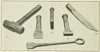
Fig. 131.—Tools used in calking with sal ammoniac and iron filings the joints of an iron-lined tunnel. (Courtesy of *Pennsylvania Railroad*.)
