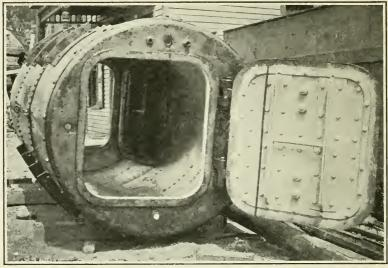
Fig. 98.—An air lock. The angles riveted on the outside are to anchor the lock in the masonry bulkhead. (Ravenswood Tunnel, A-8.)
