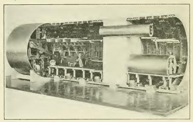
Fig. 102.—Sectional view of model of compressed air tunnel (A-18) looking toward rear of shield. (Courtesy of Pennsylvania Railroad.)
