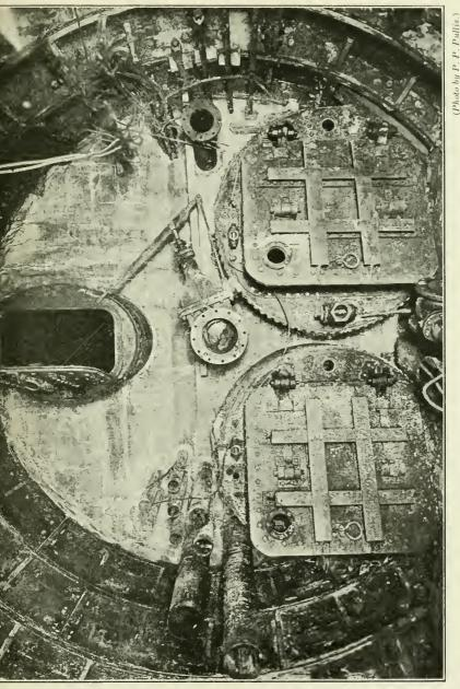
Fro. 100.—An air-lock bulkhead wall. The pressure side. Emergency lock at top. Pipe lock in middle. Man and material locks below. Air, water, electric, cable and other pipes shown. (Courtesy of New York Transit Commission.)
