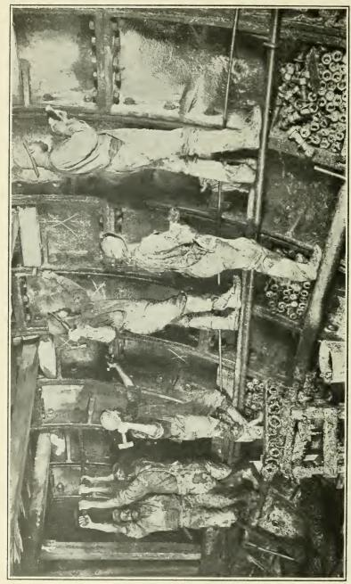
Fig. 133.—Calking and grummeting the side of an iron-lined tunnel. Pennsylvania Railroad Hudson River Tunnels, New York (A-18). (Courtesy of Pennsylvania Railroad).
