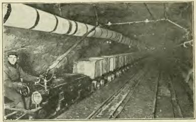
Fig. 88.—Electric locomotive with overhead trolley wire in tunnel. (Courtesy of Hudson and Manhattan Railroad.)
