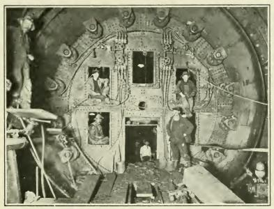
Fig 57.—Rear view of shield with erector removed. (Courtesy of Hudson and Manhattan Railroad.)
