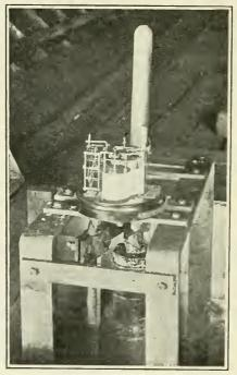
Fig. 137.—A recording gauge in the invert of a tunnel. This gauge records the movement of the tunnel in relation to a fixed vertical rod passing through the bottom of the tunnel, and having its lower end wedged in the bed rock below. (Courtesy of *Pennsylvania Railroad*.)
