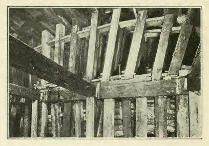
Fig. 6.—English timbering, showing bars, props, sill and stretchers. City and South London Railway (E-10).
