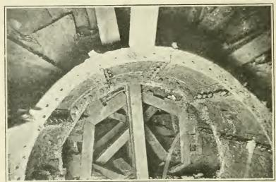
Fig. 127 A.—Haskin's Hudson Tunnel (A-6). Some of his wrought iron lining plates uncovered during the construction of the uptown tunnel of the Hudson and Manhattan Railroad (A-17).
