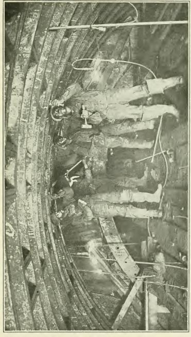
Fig. 132.—Calking and grummeting in the roof of an iron-lined tunnel. Pennsylvania Railroad Hudson River Tunnels, New York (A-18). (Courtesy of Pennsylvania Railroad.)
