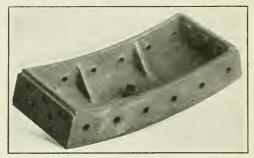
Fig. 28.—One segment of a cast iron lining.
